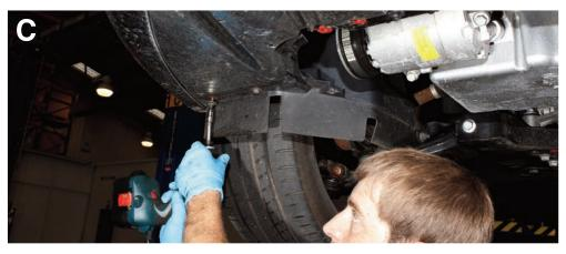
STEP 7: Undo the two bumper bolts (by headlights). Then unclip the front bumper from the wing on both sides
